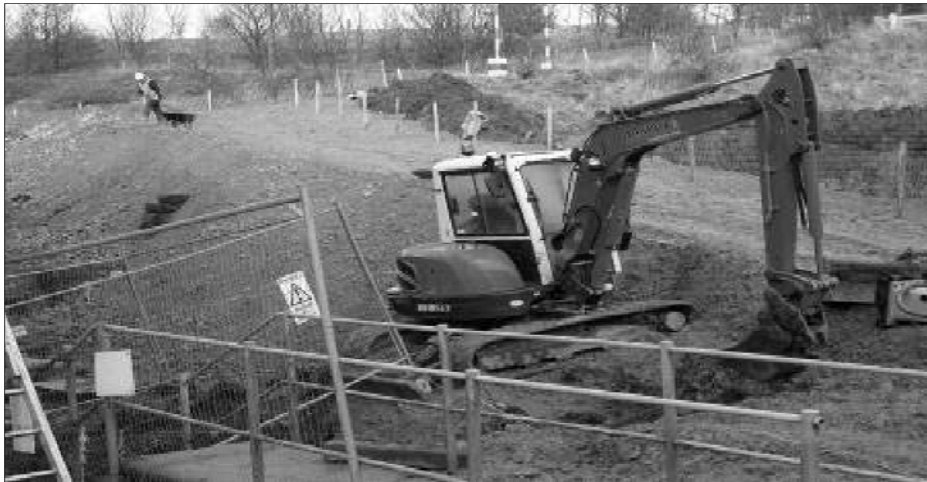
Figure 6. Construction of temporary access track across embankment
