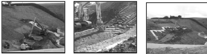
Figure 10. Placing Filter and Embankment Stability Works
