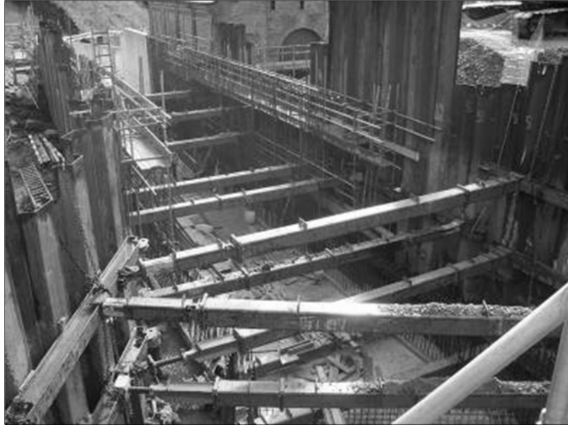
Figure 7. Phase 1 Temporary works adjacent to pump house
