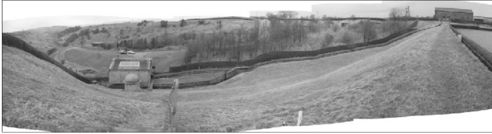
Figure 1. Panoramic view of the existing embankment with lower Coldwell Reservoir to the right and the existing pump house at the toe of the embankment.
