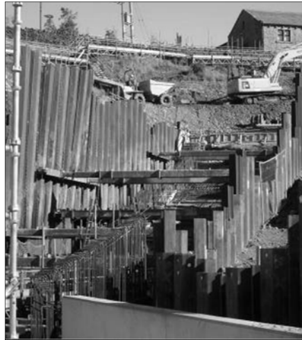
Figure 8. Phase 2 Temporary Works along new spillway chute
