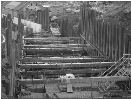
Figure 8. Phase 2 Temporary Works along new spillway chute
