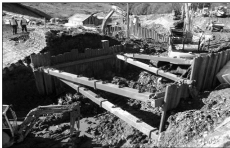
Figure 9. Phase 3 Temporary Works for crest bridge and tumble bay
